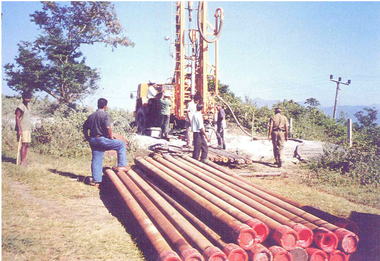
The GSN Station PALK 100m, steel-cased, Borehole
