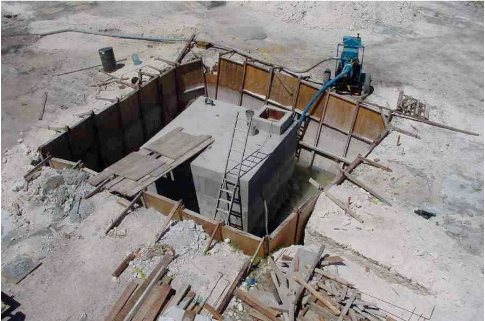
DGAR - vault under construction
