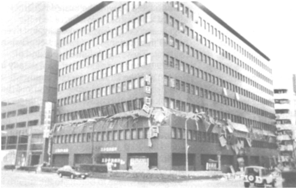
Figure 0: Story collapse in a modern building in the Sannomiya district of downtown Kobe. Photograph by Paul Somerville.
