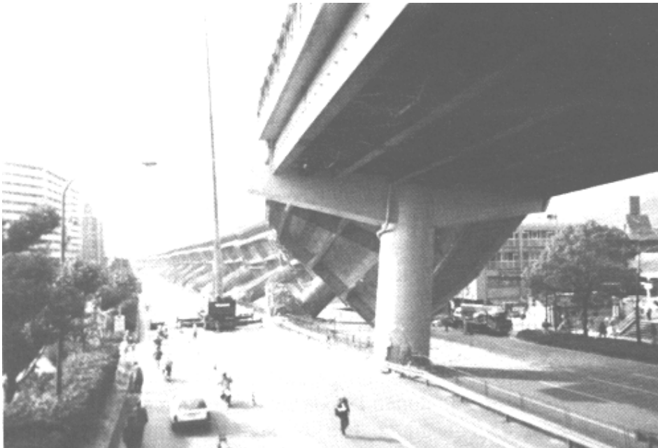
Figure 0: Collapse of the Hanshin Expressway in Nishinomiya. Photograph by Paul Somerville.
