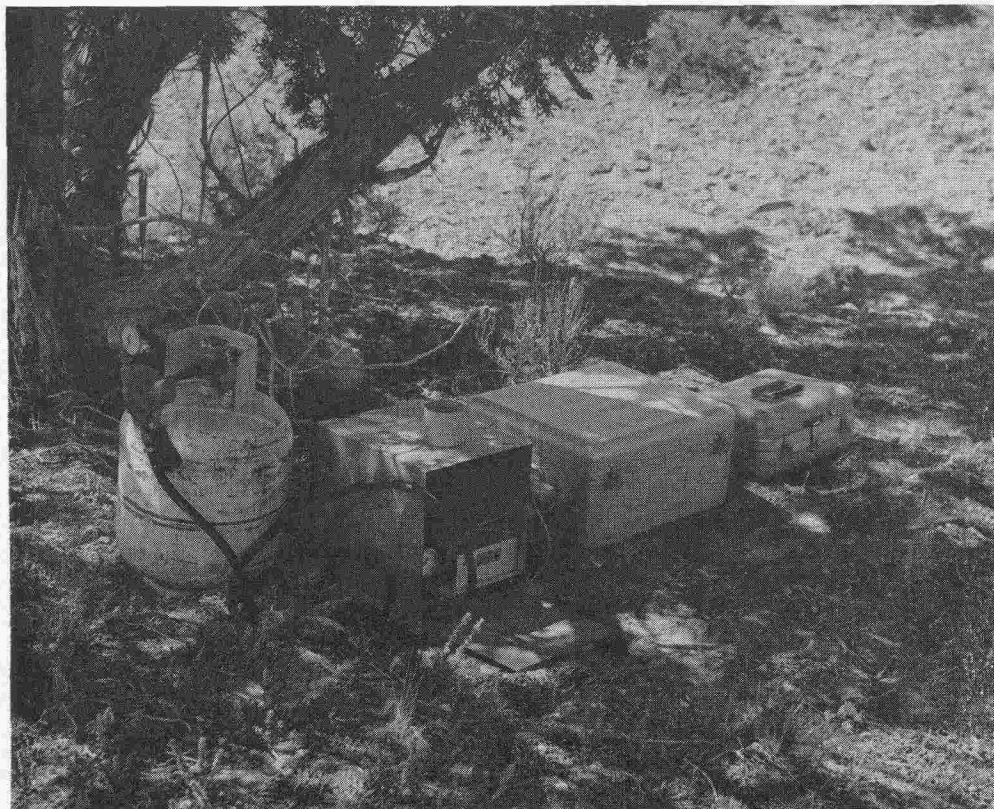
FIG. 3. Portable seismograph station. The units shown in the photograph are, left to right : propane tank, thermoelectric generator, 12-v battery, tape recorder, seismic amplifier. The antenna and seismometers are not in the picture.
