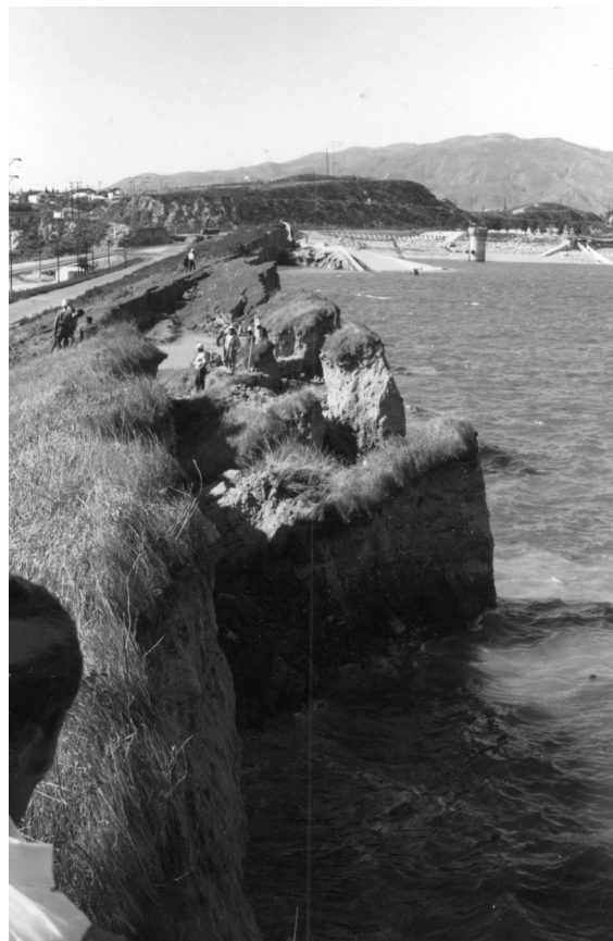
Figure 1. Remains of crest of Lower San Fernando Dam, damaged by a landslide following the magnitude 6.5 earthquake of February 9, 1971. Men on left are looking down at reservoir water, which is only 1.4 m below them. One outlet tower is visible in the right background; the other tower was knocked down by the landslide and was submerged in the reservoir. Photograph by T. L. Youd, U.S. Geological Survey, February 9, 1971.
