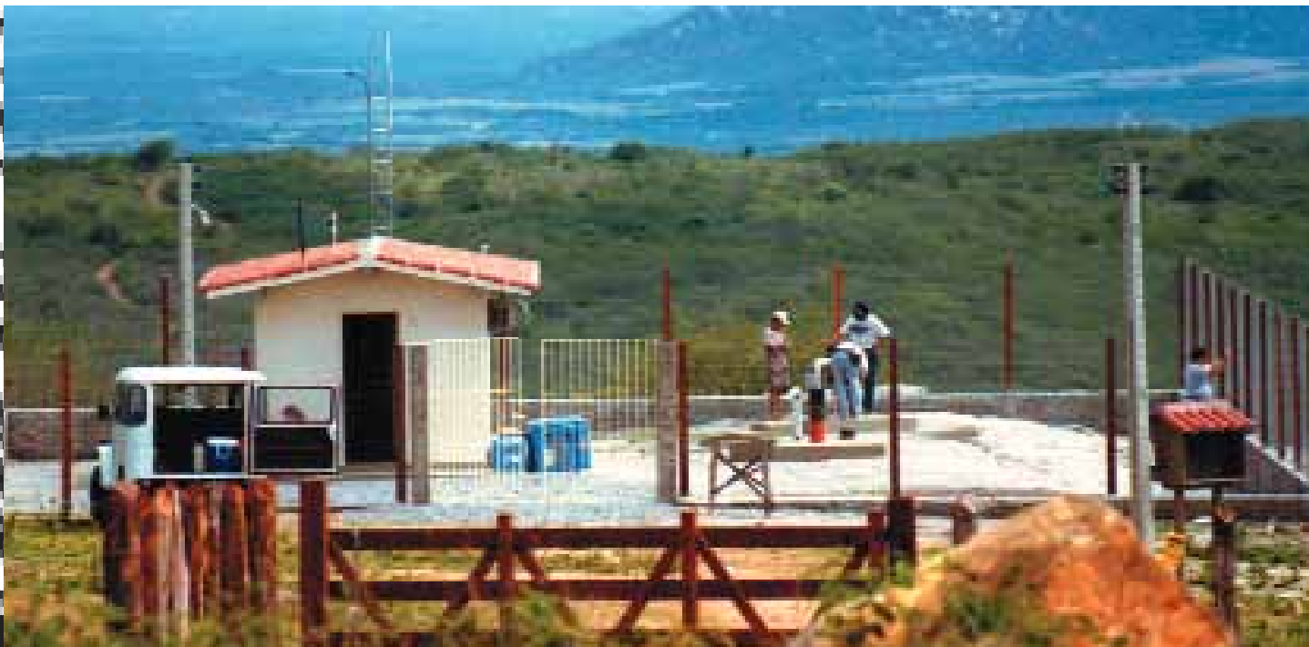
Above: Finishing touches are being made at the borehole wellhead for a new GSN site in northeastern Brazil—Riachuelo, RCBR. The GSN equipment was installed by a USGS, Albuquerque Seismological Laboratory field team in March of this year. Broadband borehole sensors are installed at depths of 100 meters and 40 meters. There is also a low-gain sensor installed at the surface.
