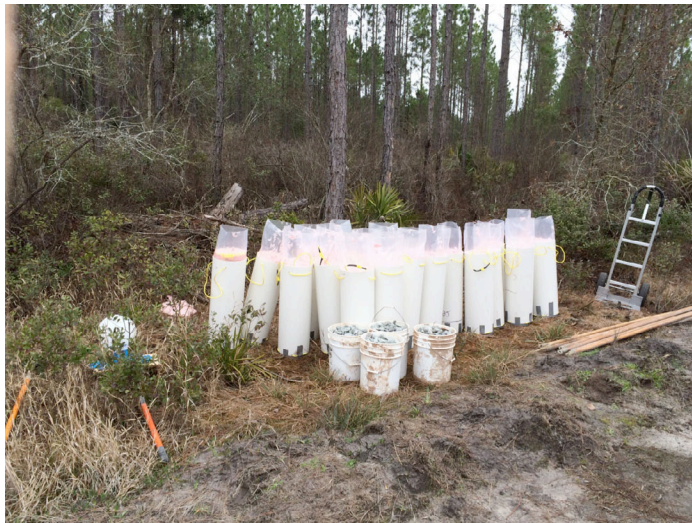
Fig. 6: Emulsion filled cartridges being prepared for loading at L1-14.
