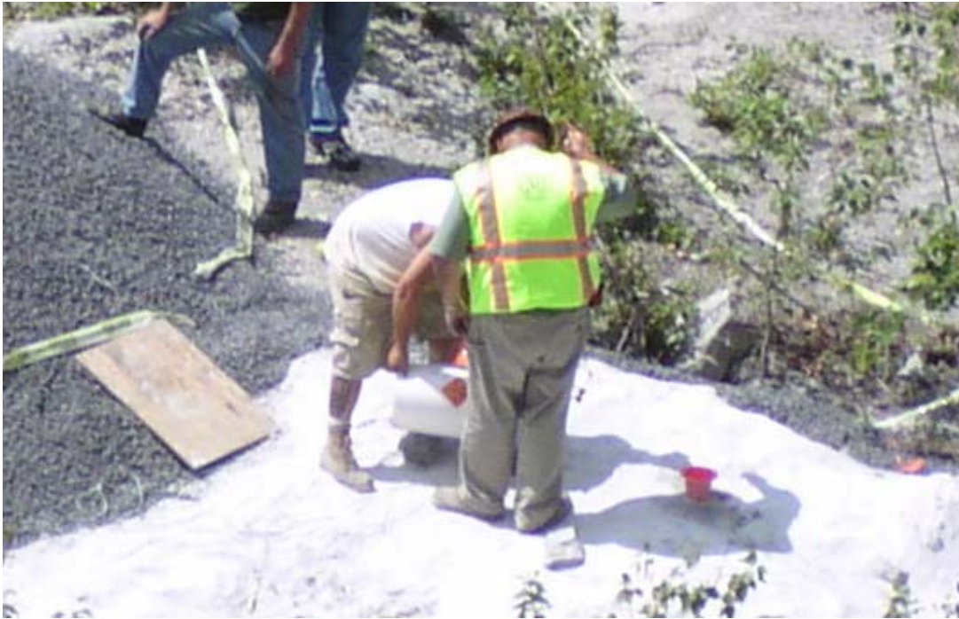
Figure 15. Loading of ANFO/Emulsion explosive.
