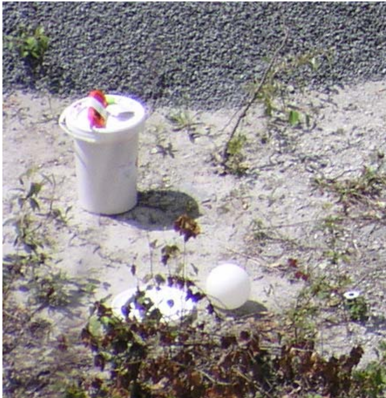
Figure 18. Blast plug (white ball) used to help stem the holes.
