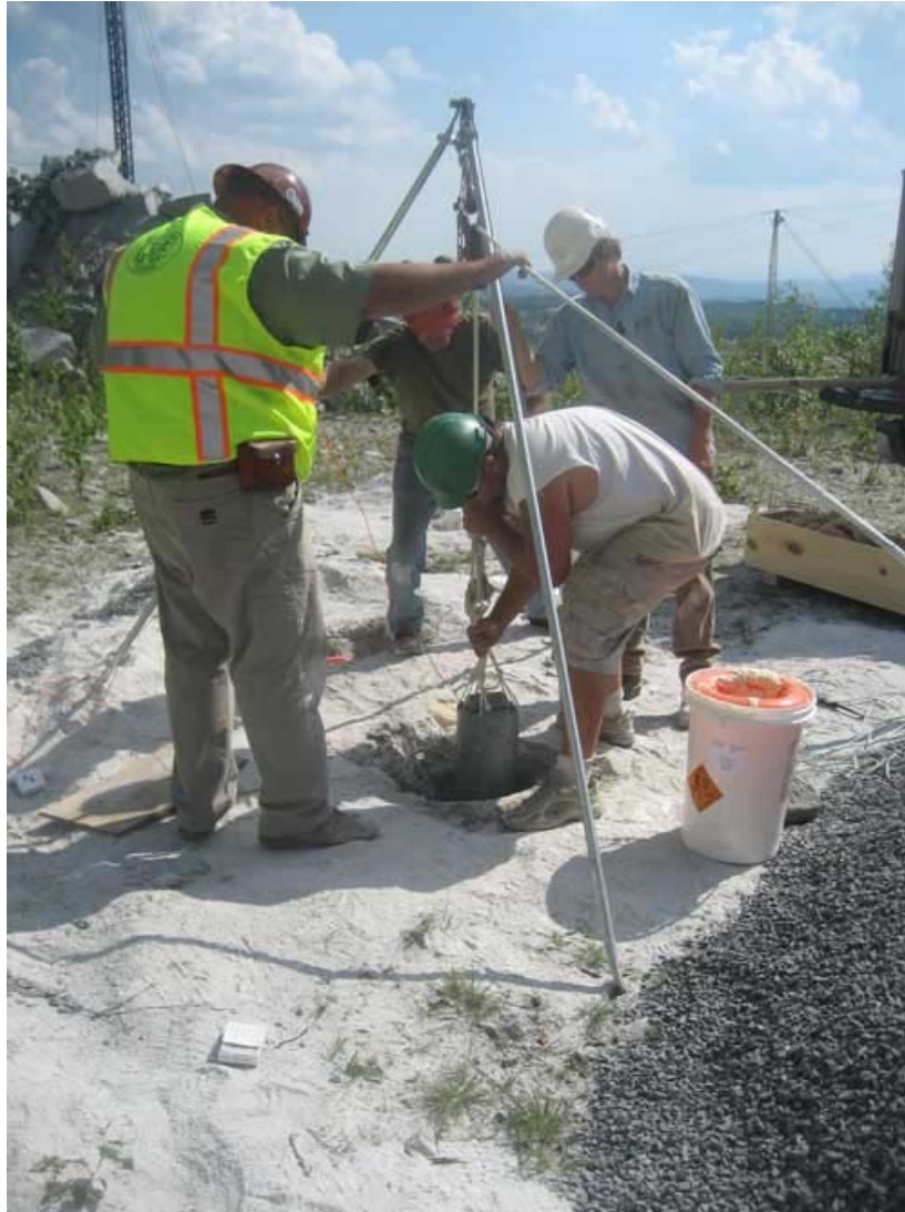
Figure 17. Lowering the COMP B charge into the hole.
