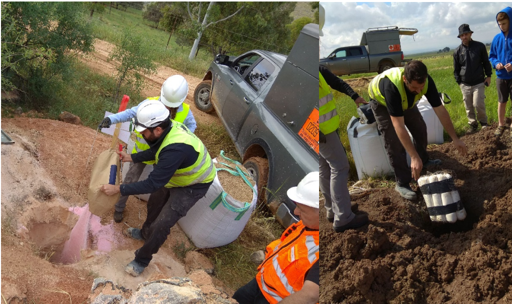
Figure 7 – Explosives load: Anfo type explosive (left), and emulsion type (right).
